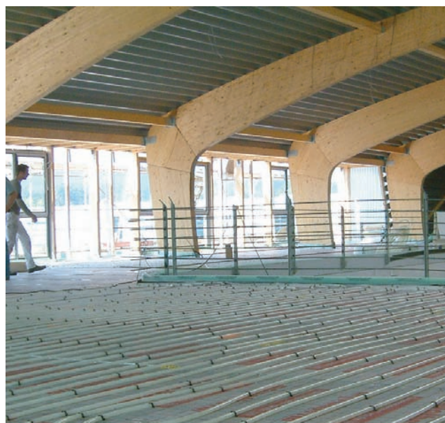
MAX-FITNESS-CENTER, Installing of sports floor heating system
