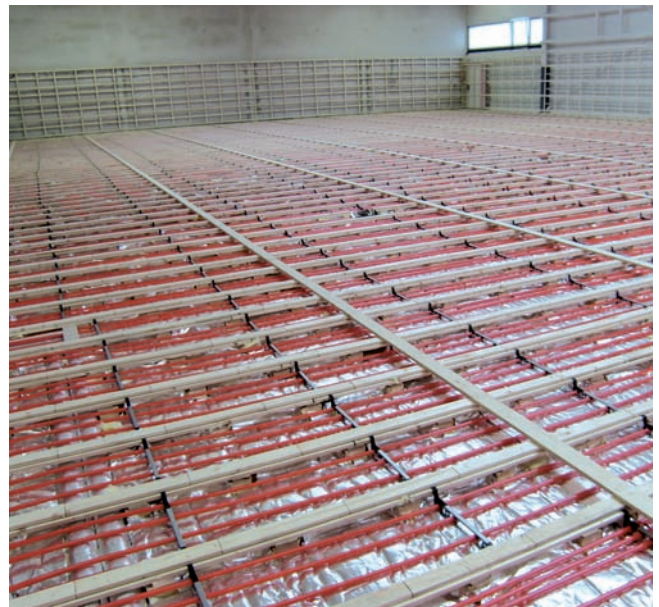
aquatherm® sports floor heating system.
