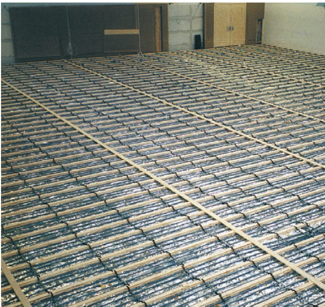
Installation technique with pipe guiding rail.
