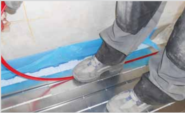
Laying of heating pipes
