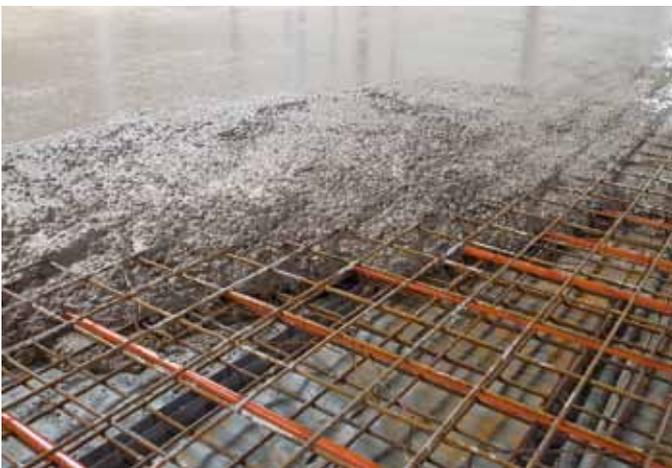
**AQUATHERM INDUSTRIAL SURFACE HEATING (FUNCTIONAL HEATING)**
